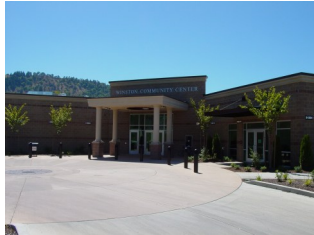
Main Entry Portico
