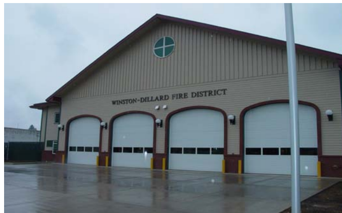
Front of Apparatus Bays
